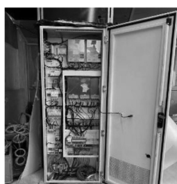
Fig. 7. The DC instrument cabinet at site.
