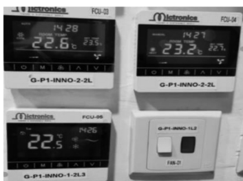
Fig. 8. Loading control panels of the fan coil units.
